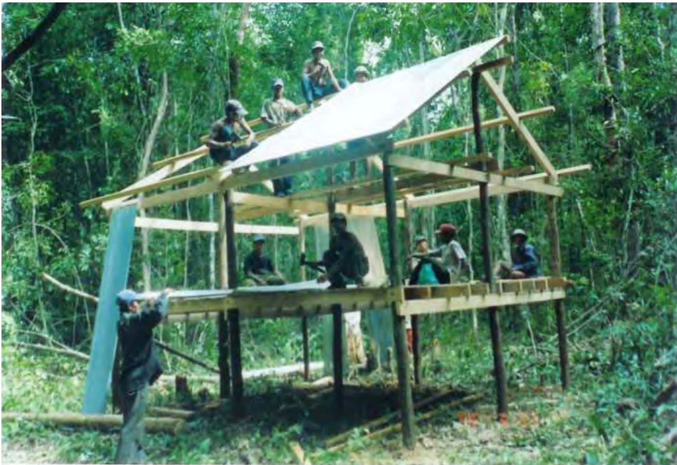
Villagers in Dong Kombut CF construct a patrol post.
